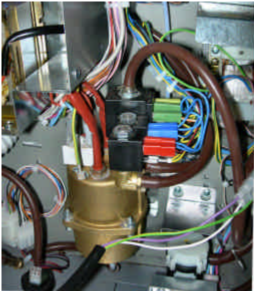
LOCATION OF PRESSURE BOILER
